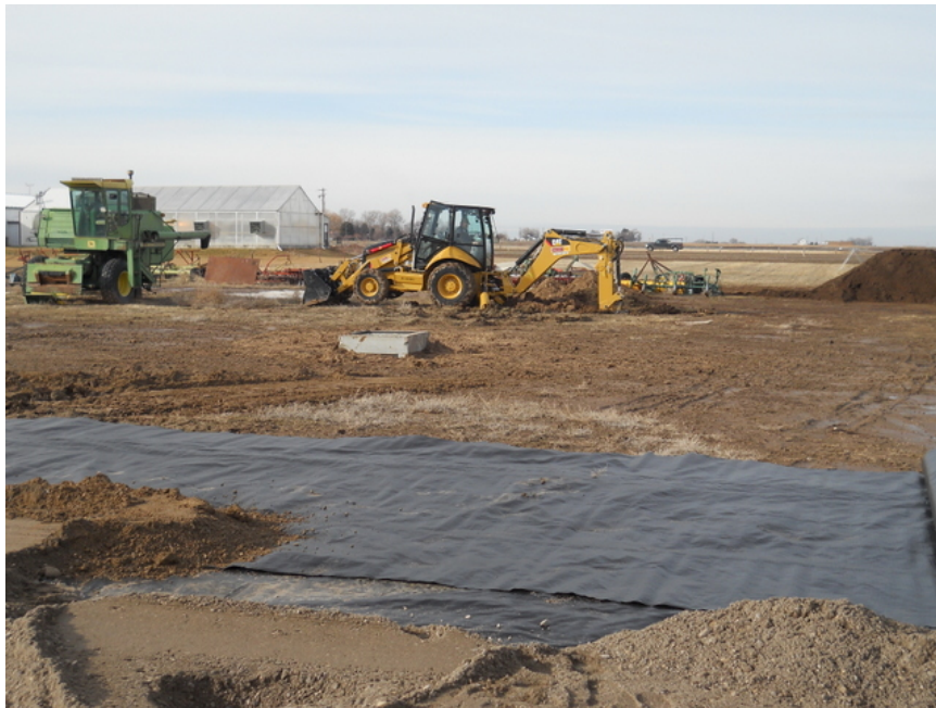
Figure 7-13. Kimberly site preparation.
