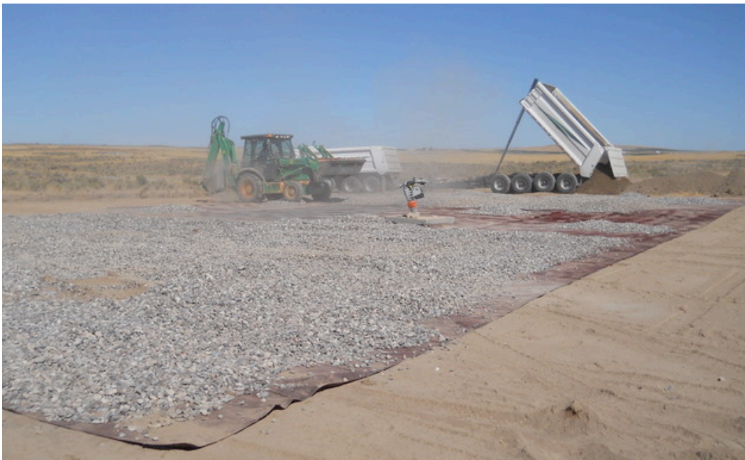
Figure 7-4. Kimama site preparation.
